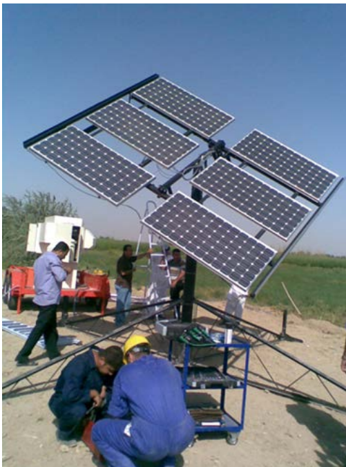
The tracking solar array provides maximum power, following the movements of the sun.
